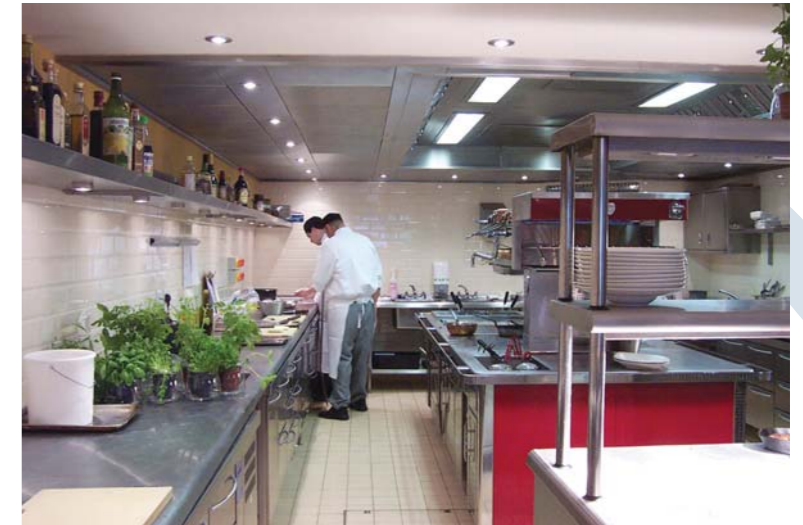
Integrated Kitchen Ventilation Ceiling System Reducing the fire risk in your kitchen.
