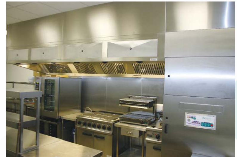
The self contained kitchen ventilation system that needs no direct ductwork connections to atmosphere
