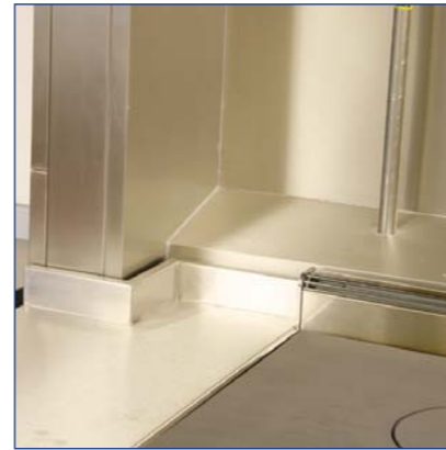
Above: close up detail of splashback cladding working around services pipework and support frame. Left and below: wall canopy showing the ground support frames and supply air diffusers.
