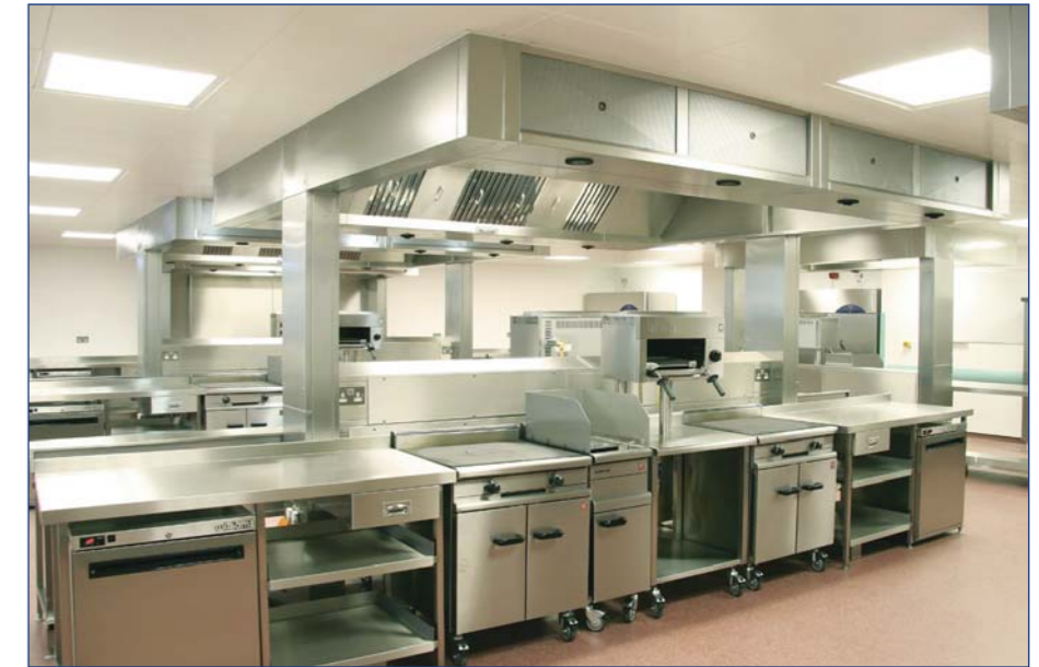
Above: close up detail of service distribution unit that works around structural column and support frame. Right and below: Island canopy showing the ground support frames, supply air diffusers and ductwork connections.
