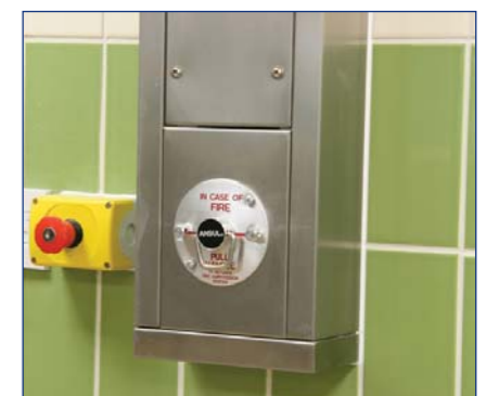
Some canopies on the project, were also protected with fire suppression systems. At the request of the project architect, Britannia manufactured special housings for the manual pull activation systems, to ensure an easily cleanable hygienic kitchen.
