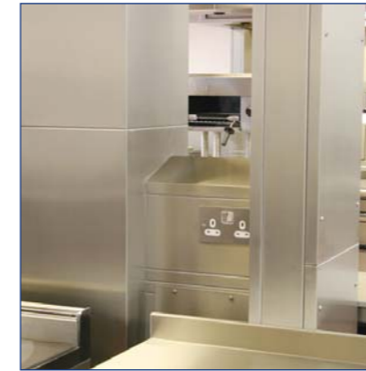
Above: close up detail of service distribution unit that works around structural column and support frame. Right and below: Island canopy showing the ground support frames, supply air diffusers and ductwork connections.
