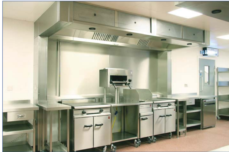
Above: close up detail of splashback cladding working around services pipework and support frame. Left and below: wall canopy showing the ground support frames and supply air diffusers.
