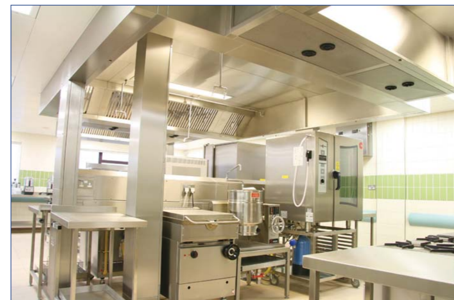
Some canopies on the project, were also protected with fire suppression systems. At the request of the project architect, Britannia manufactured special housings for the manual pull activation systems, to ensure an easily cleanable hygienic kitchen.
