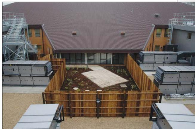
A project with so many kitchens requires extensive air movement facilities. The central courtyard at Worthy Down is packed with the very latest air handling units to handle both extract and supply from 14 kitchens.
