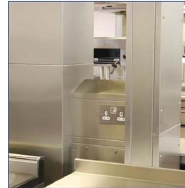
**Above:** close up detail of service distribution unit that works around structural column and support frame.
