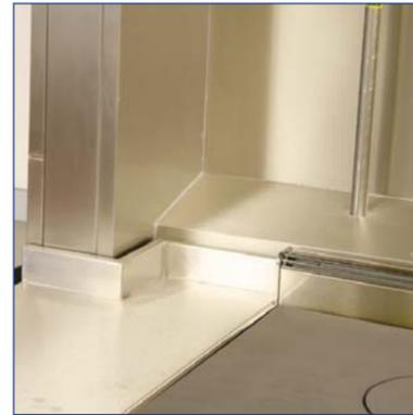
**Above:** close up detail of splashback cladding working around services pipework and support frame.
