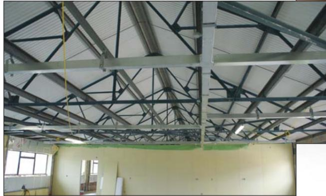
The existing fragile roof structure was only able to support its own weight. As a result it was necessary to incorporate ground support frames when installing the ventilation canopies.
