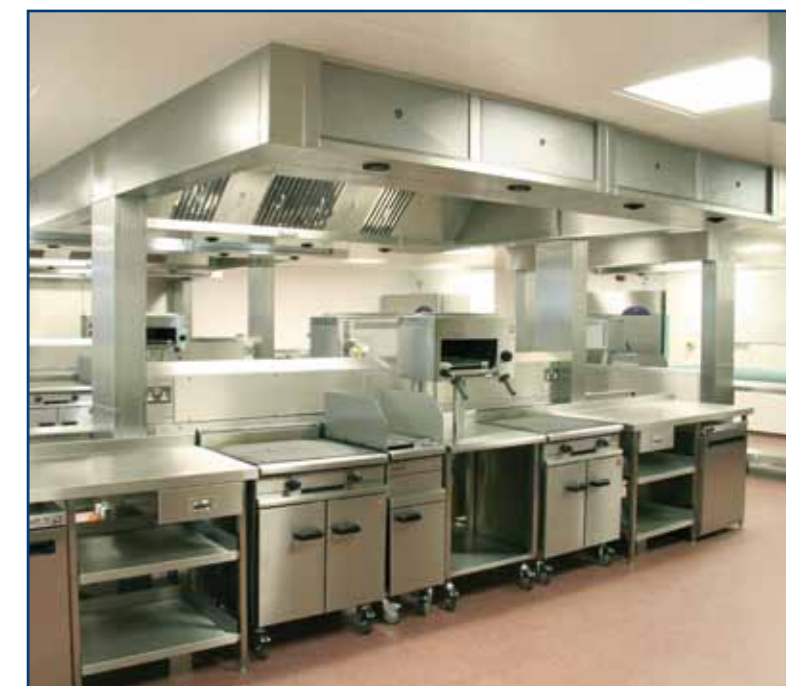
Econex canopies installed at MOD Catering School, Worthy Down.
