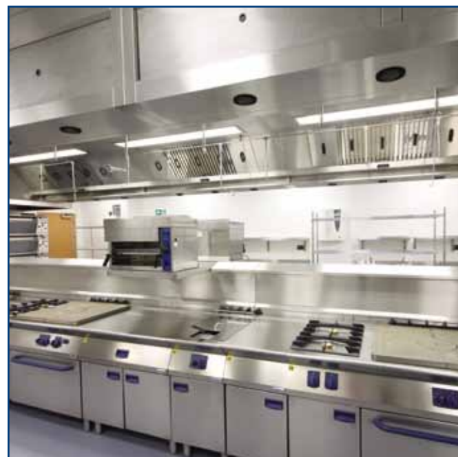
Econex canopies installed at South Bristol Skills Academy
